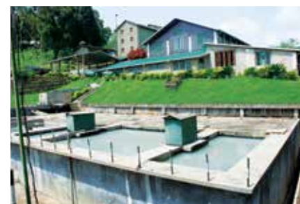
Effluent treatment plant - Panawatte
